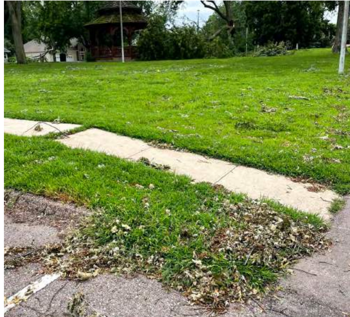
ASPHALT DRIVE SIDEWALK APPROACHES
