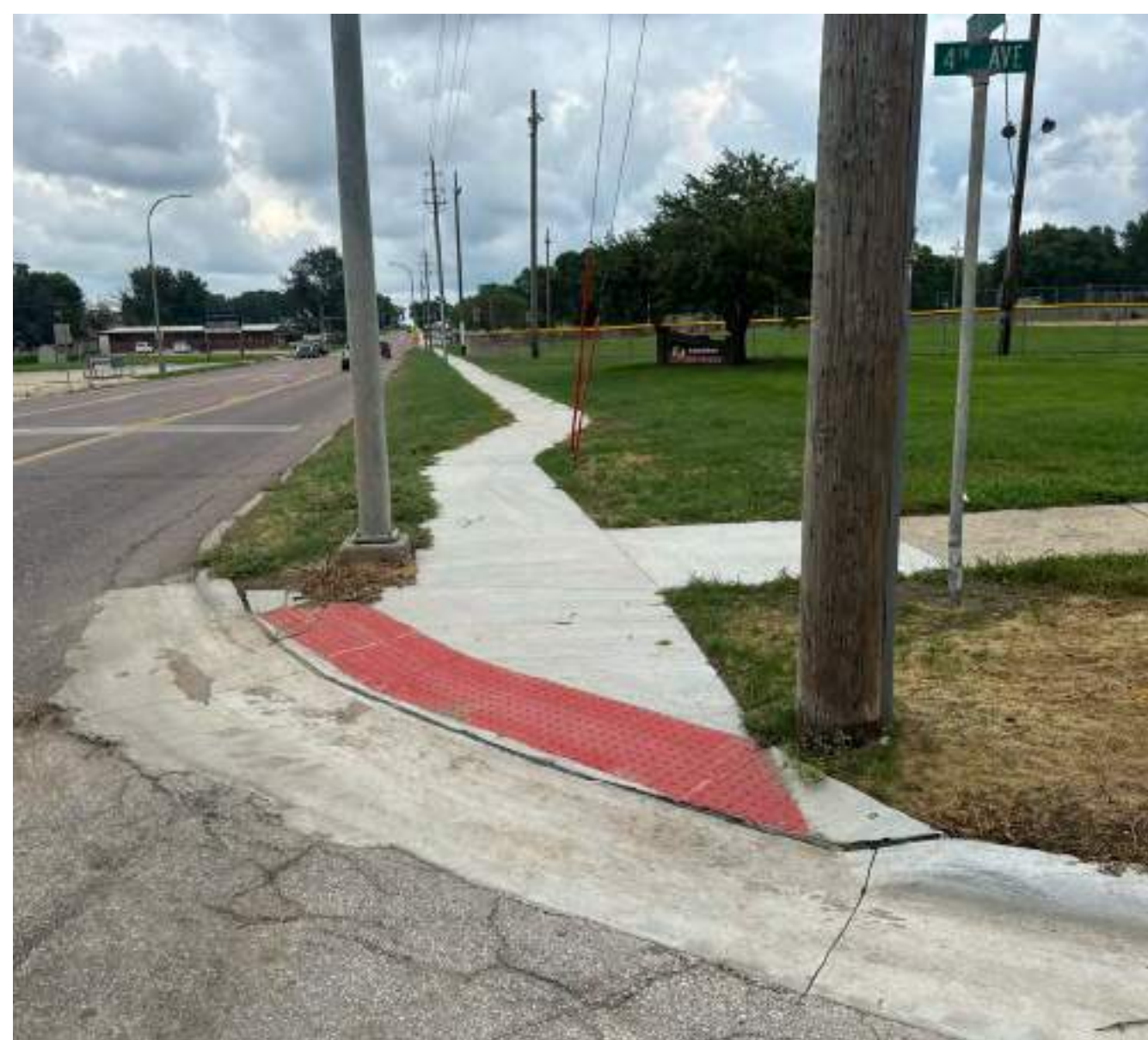
320TH STREET SIDEWALK
