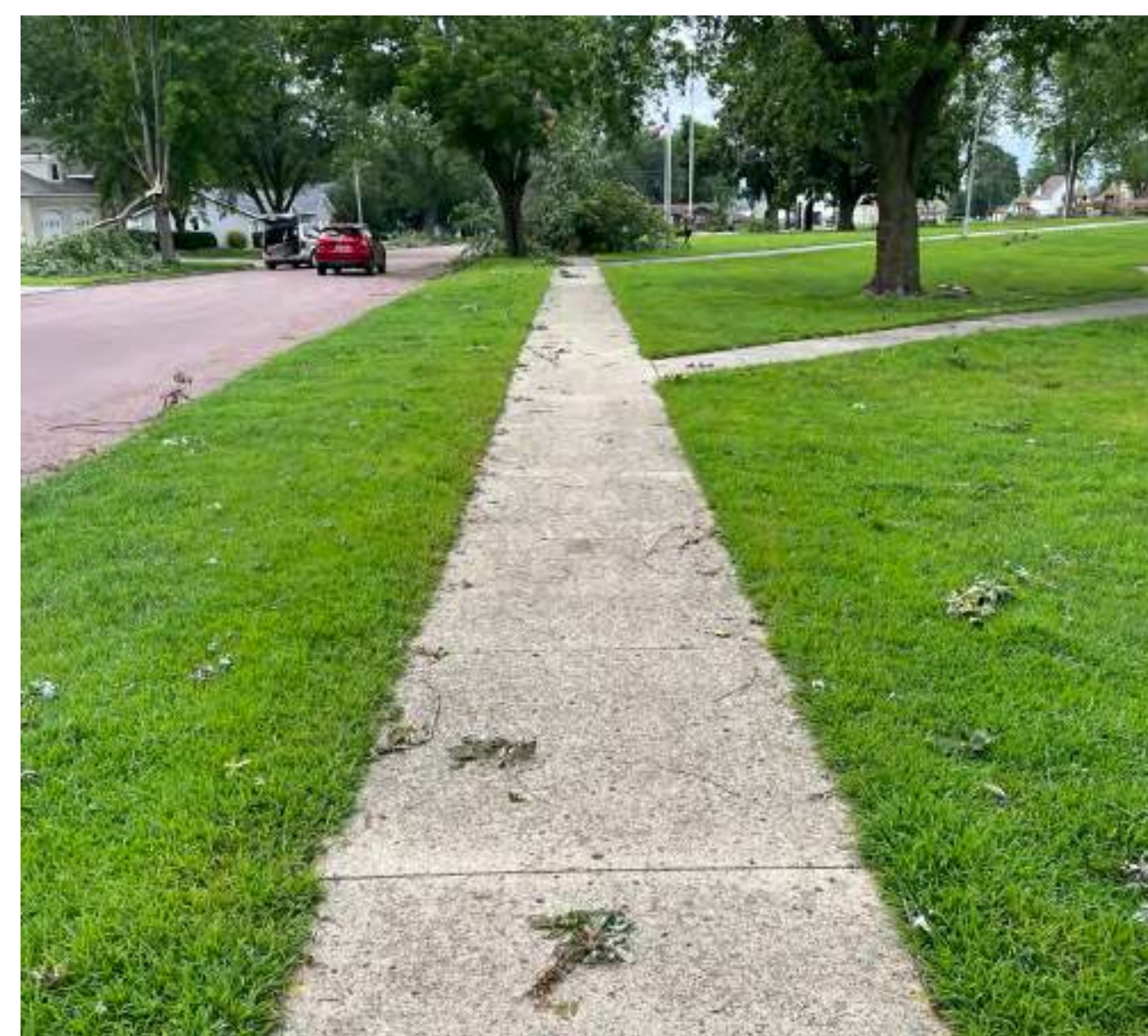
6TH STREET SIDEWALK
