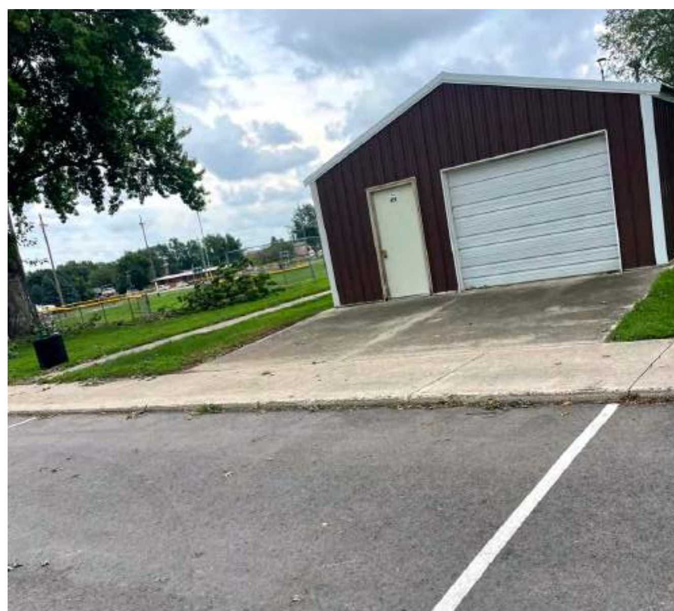
WEST GARAGE DRIVEWAY
