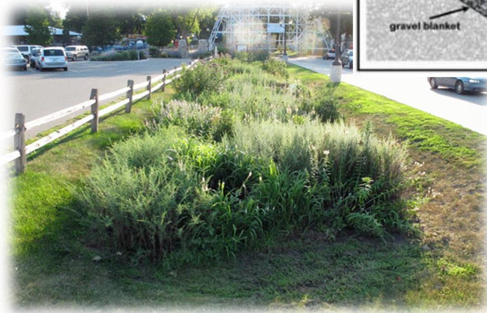
**Bioswales** – This form of low impact development is similar to a rain garden in its objective, but instead of a strategically placed depression to collect water, Bioswales are a designed conveyance system to collect and move water in lieu of storm sewers. Bioswales improve water quality by filtering the first large push of storm water after a large rain event.
