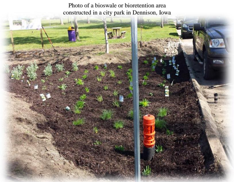
Photo of a bioswale or bioretention area constructed in a city park in Dennison, Iowa
